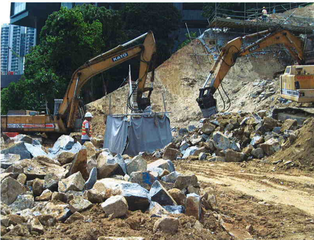
2. Sound insulation sheet surrounding the rock breaking activities as far as possible.
