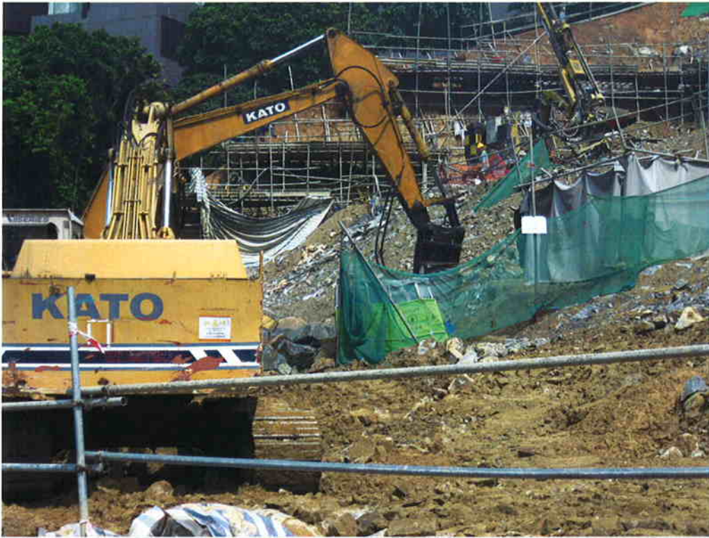
3. Noise insulation material for rock breaking.
