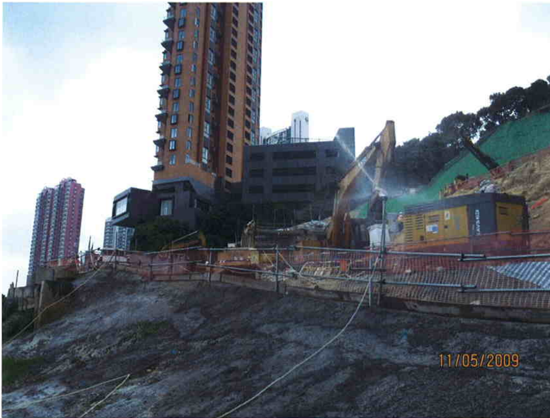
2. Automatic sprinkler spraying the haul road.
