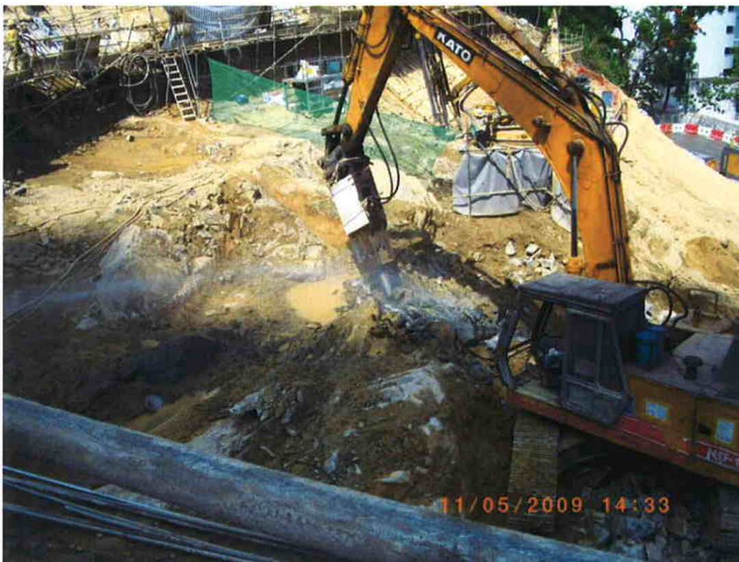
3. Water spraying during rock breaking.
